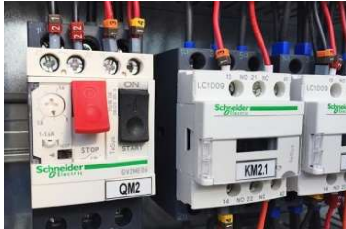
Figure 2. Thermal Overload Relay (TOR)
