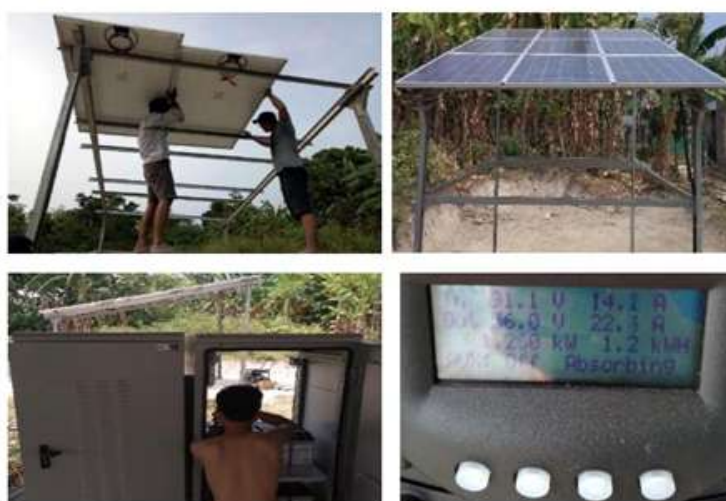
Figure 2. Installation of solar modules
