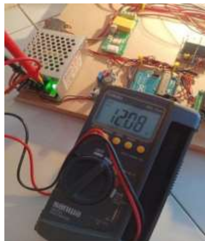
Figure 9. Power Supply Output Testing
